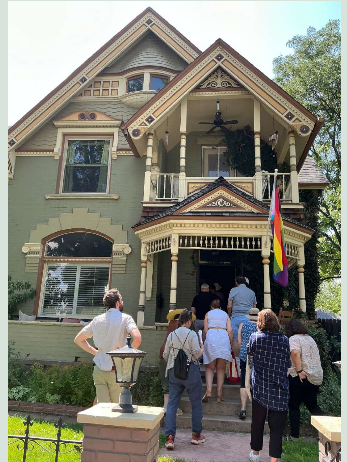
Housing cooperative, Colorado
